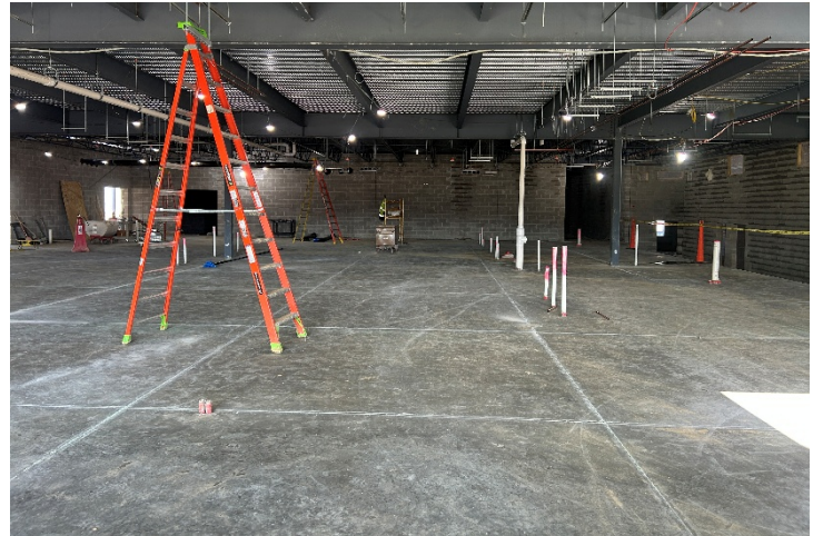
Slab on Grade Finish Work in the Administration Space
